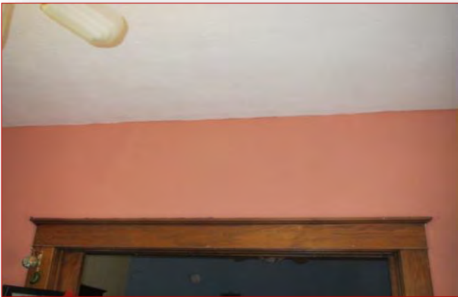
Figure 2 Notice how much wall you have above the existing header. This header is diffusing a lot of weight. Also notice how large the posts are or how much wall there is to each side of the existing header. Great care in selecting a suitable LVL to distribute this new weight is essential. There are online calculators available that determine the size you need to create a more inviting open space.
