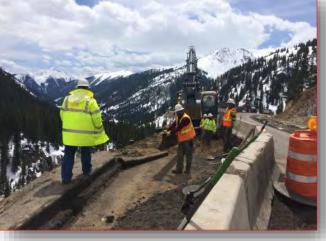
Crews use heavy equipment to guide a new beam into place which will ultimately strengthen the crib wall (retaining wall) underneath the highway. Courtesy photo.
