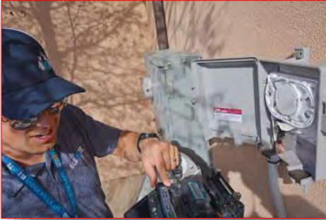
Dakota Cole, Elevate fiber optic specialist, connects the live exterior fiber cable to the home fiber cable using a fusion splicer. The equipment on the outside of the home, called a demarcation box, will protect this connection and serve as a convenient location for troubleshooting if the need arises. Photo by Phil Sanchez, DMEA communications specialist.
