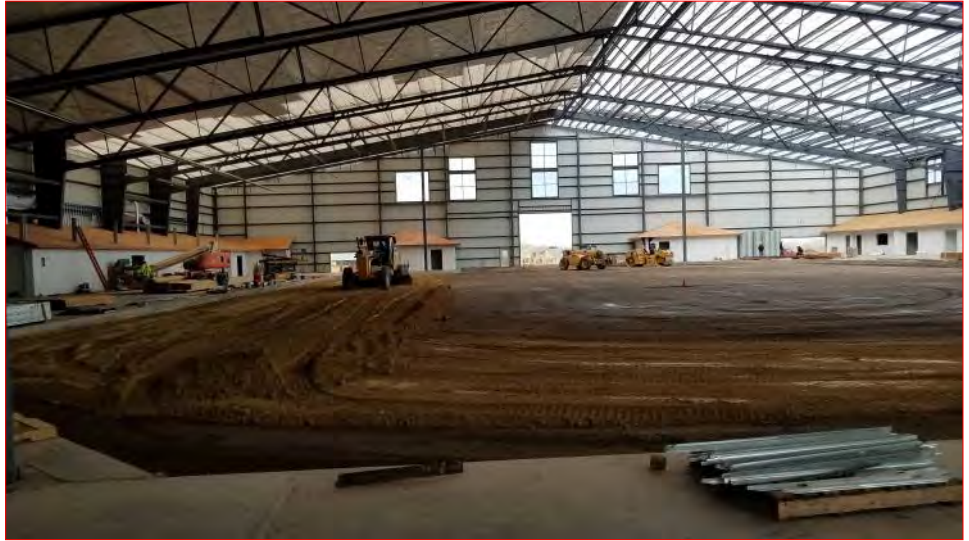
On Nov. 29, 2017 local clay was brought in and compacted for the Event Center arena floor. Photo by Gail Marvel.
