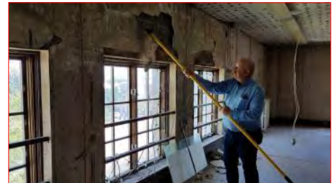
Board of County Commissioners (BOCC) Chair Keith Caddy easily dislodges plaster that no longer adheres to the walls of the third-floor of the Montrose County Court House. Photo by Gail Marvel.
