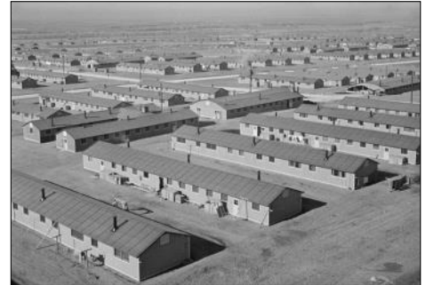
The Amache incarceration site in Colorado, Dec. 12, 1942. Among the new grant projects, Colorado Preservation, Inc., will develop interpretive elements at the site to provide visitors with a better understanding of Japanese American incarcerated living conditions during World War II. Courtesy photo.
