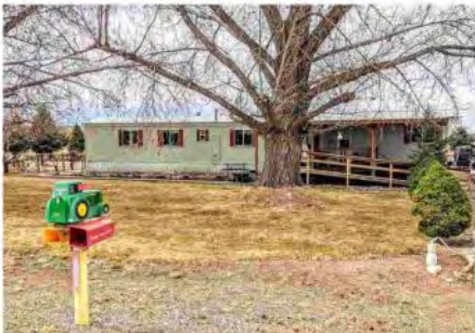
6031 5800 Road Olathe, CO Completely remodeled!
