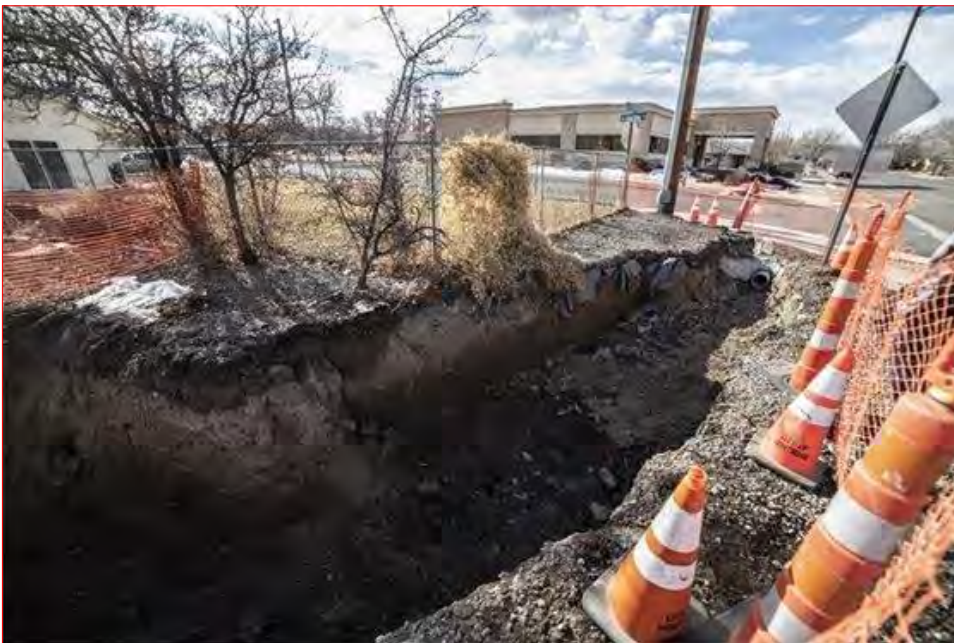
A sinkhole has developed as the result of a collapsed storm drain at the southeast corner of South 5th Street and Junction Avenue. Courtesy photos City of Montrose.
