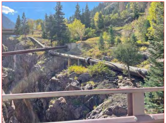
The large pipe, seen here just above the bridge near the Box Canyon entrance, carried water to the Ouray power plant. A few hundred feet below the bridge the pipe crosses the canyon. The power plant is located just below the south end of Oak Street. Photo by Bob Cox
