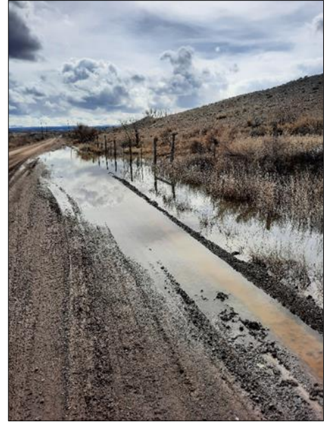
Damage to County Road 5960 from mesa run-off below the current 10-acre gravel pit.
