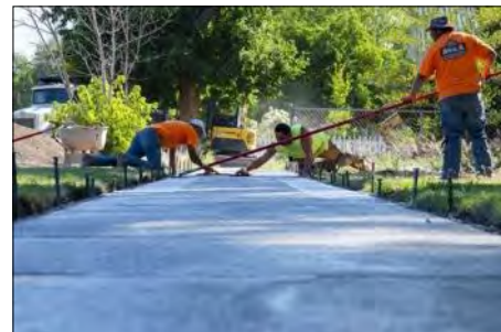
Workers with Avila Concrete, a contractor working for the City of Montrose, smooth out a fresh concrete sidewalk poured along the 100 block of South Fourth Street in downtown Montrose. City of Montrose courtesy photo.
