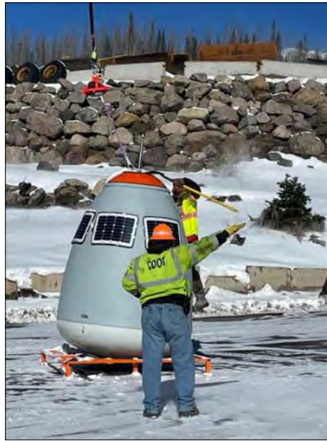
Each winter CDOT crews reset O'bellx units onto fixed and permanent bases on US 160 Wolf Creek Pass, in Mineral County. Courtesy photo.
