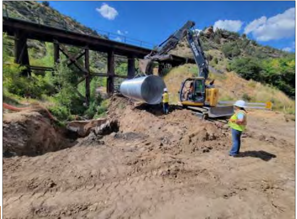
Excavation and placement of the new 72" culvert pipe at Mile Point 16 on CO 133. Courtesy photo.
