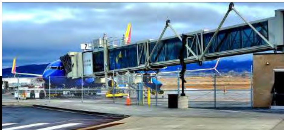
installed as a part of the airport's recently completed additions, upgrades, and remodeling of the main terminal building. The addition of the two new jet bridges at gates 6 & 7 mean that passengers no longer have to enplane and deplane through outside stairs and are now protected from the elements," White said.
